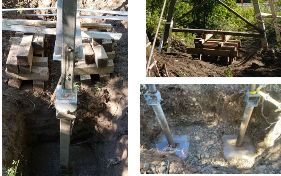
Figure 6: A-frame footings installation of additional base plate
