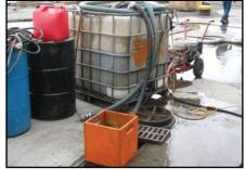
The trench drain is blocked and a sump pump is installed to collect wash water into a tote.
