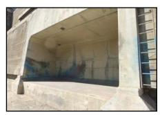
Paint overspray due to INADEQUATE containment stablizer pocket doors.
