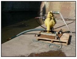
The sill diversion pump removes clean seawater from the pool at the front of Section 1 (moon pool) and discharges into the tunnel drains through a hard pipe on the graving dock wall.
