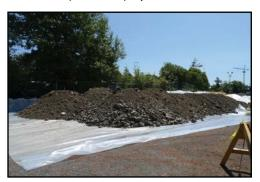
INADEQUATE stockpile of contaminated soil. Soil should be covered to prevent exposure to elements, runoff and people.
