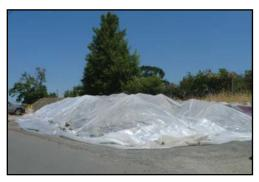
ADEQUATE soil stockpile management. Soils placed on poly and covered.
