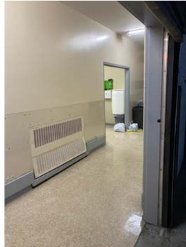
Picture 3: Picture from loading dock door looking inside loading dock area
