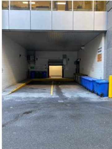
Picture 2: Loading dock 255 with door open
