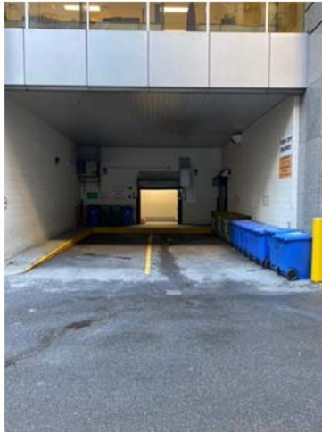
Picture 2: Loading dock 255 with door open
