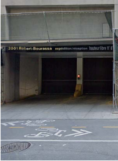
Picture 1: View of loading bay from street
