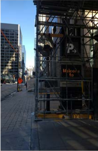
Picture 1: Picture from street of side of 121 King Street West where loading dock is located.
