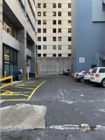
Picture 1: Picture from street of side of 255 Albert where loading dock is located.
