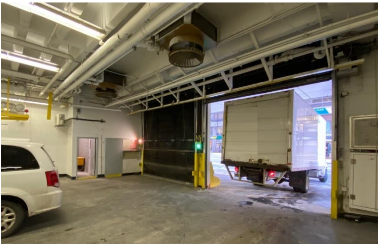
Picture 3: View of garage doors from inside
