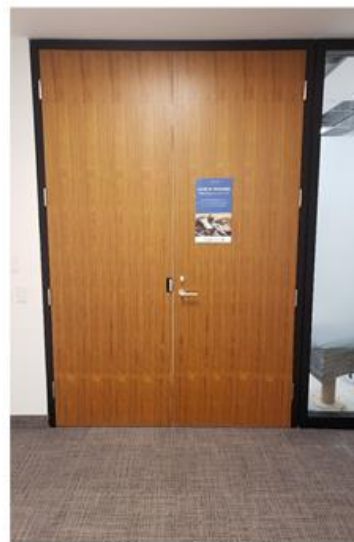
Picture 7: Picture taken from lobby of Hallway towards storage of desks
