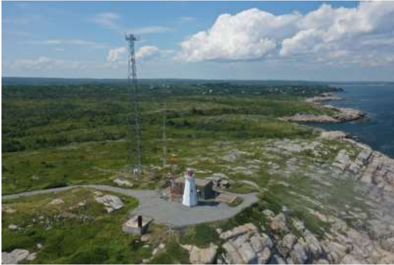
Aerial view of site looking from southeast.
