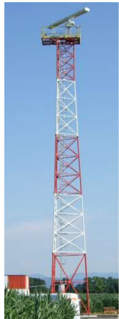
Figure 7.1 Three-legged lattice tower
