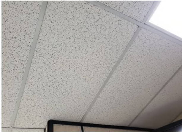
Photograph 16: Loc 4; No asbestos detected in acoustic ceiling tile 2 (2'x4' pinhole & divot)
