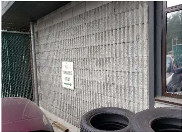
Photograph 4: Building exterior (east); wall proposed to be impacted by renovation work
