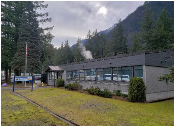
Photograph 1: Building exterior, front (north)
