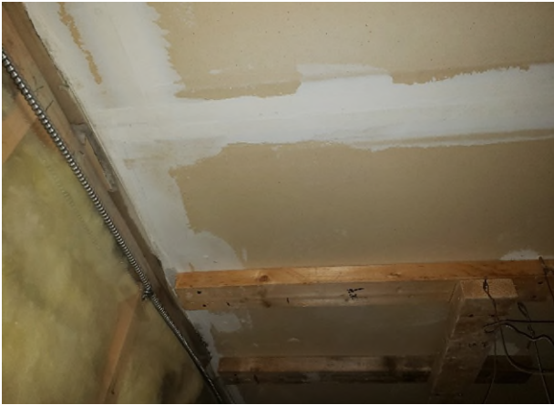
Photograph 15: Loc 1; No asbestos detected in drywall joint compound on ceiling
