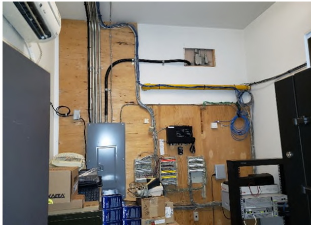
Photograph 8: Loc 2; Area proposed to be impacted by renovation work
