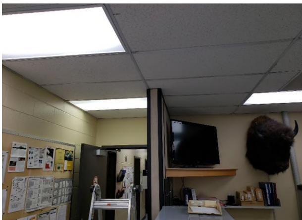
Photograph 11: Loc 5; Area proposed to be impacted by renovation work
