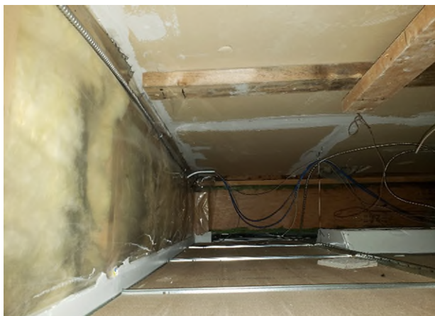
Photograph 12: Loc 1; Ceiling cavity; Area proposed to be impacted by renovation work
