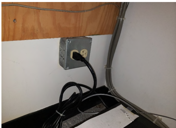
Photograph 18: Loc 2; White paint on drywall identified with lead levels that do not exceed criteria
