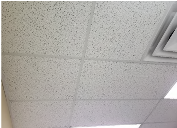
Photograph 14: Loc 1; No asbestos detected in acoustic ceiling tile 1 (2'x4' small & large pinhole)
