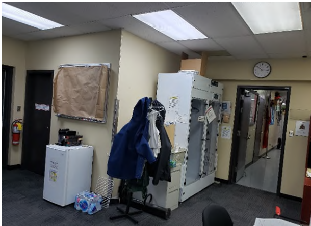
Photograph 7: Loc 1; Area proposed to be impacted by renovation work
