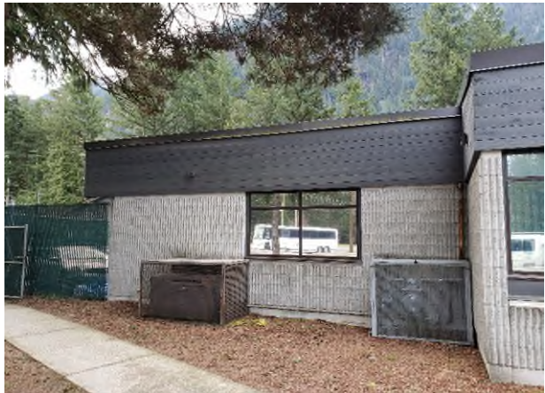
Photograph 2: Building exterior; front (north); location of old generator
