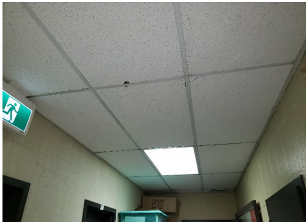
Photograph 10: Loc 4; Area proposed to be impacted by renovation work
