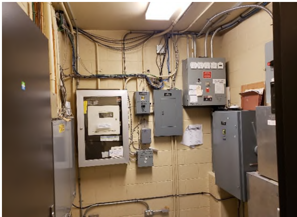
Photograph 9: Loc 3; Area proposed to be impacted by renovation work
