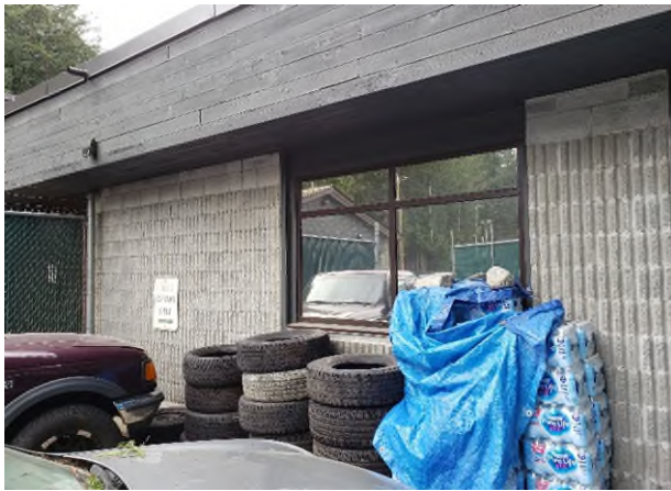
Photograph 3: Building exterior (east); location for proposed new generator
