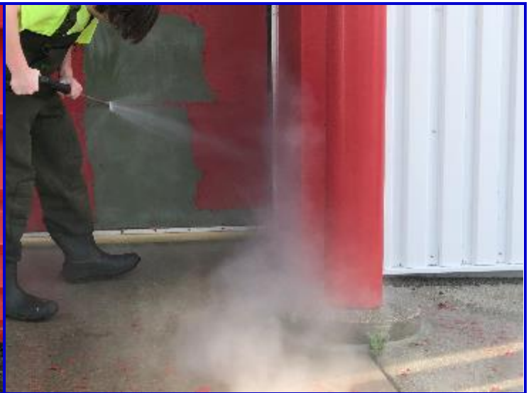
5.10 OH door powerwashing in progress
