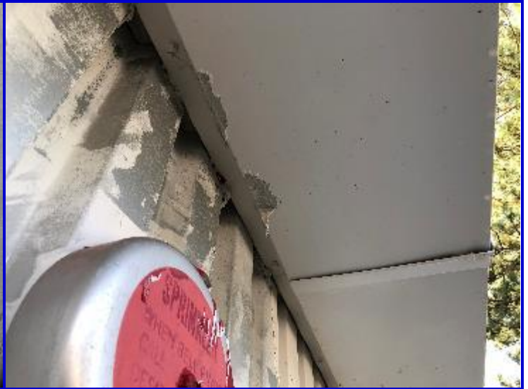
5.08 difficult removal area
