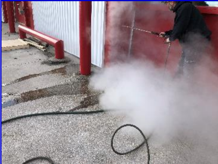
5.23 Powerwashing of door frame
