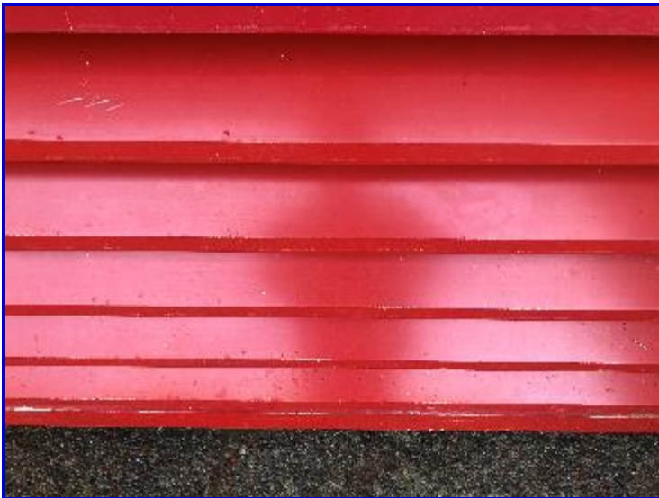
5.09 Louvre with paint removed
