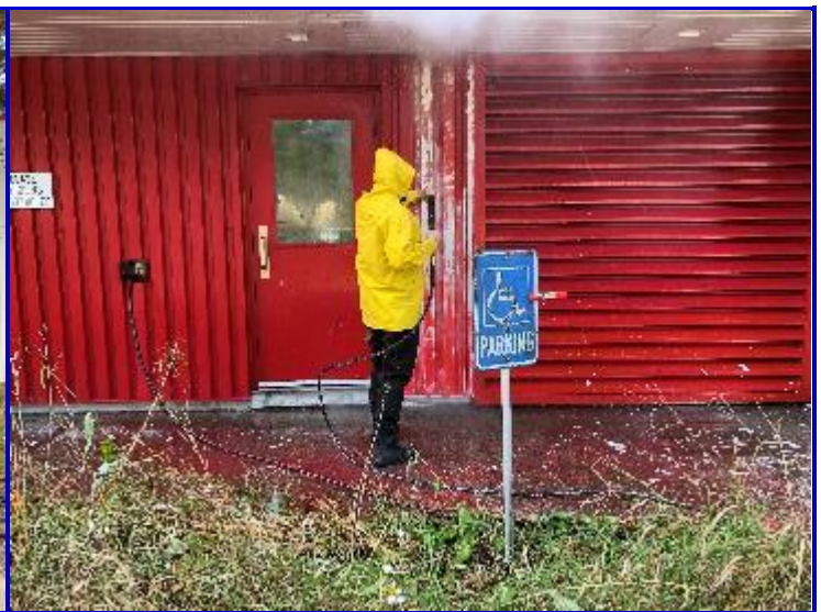
5.02 Powerwashing in progress
