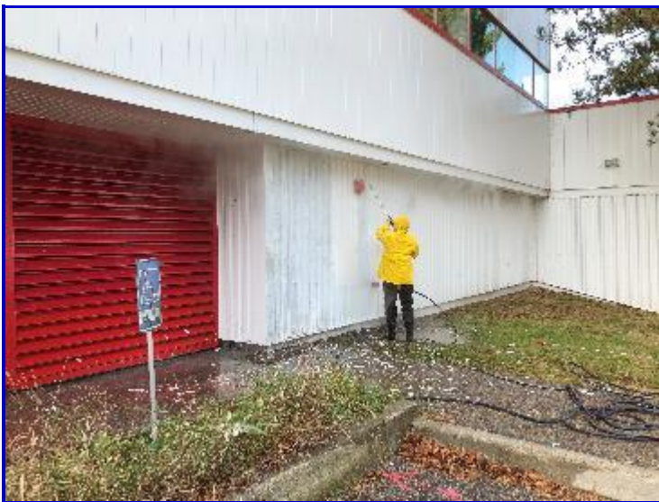
5.01 Powerwashing in progress
