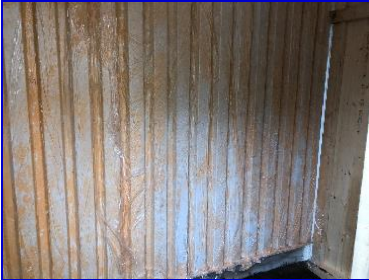
5.03 Plastic installed over the Prep220
