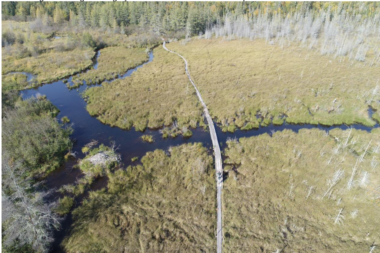
Figure 1. Aerial view of existing boardwalk structure, September 2019.
