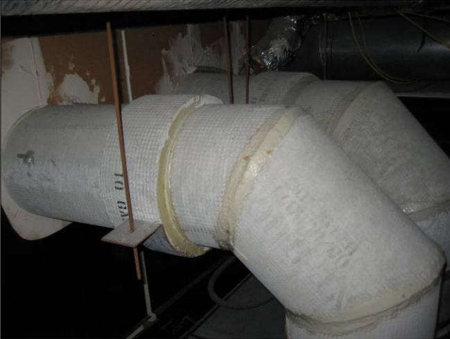
**Photograph 1:** [Room 115] Asbestos-containing Transite cement pipe vents above fume hoods observed to be in good condition.
