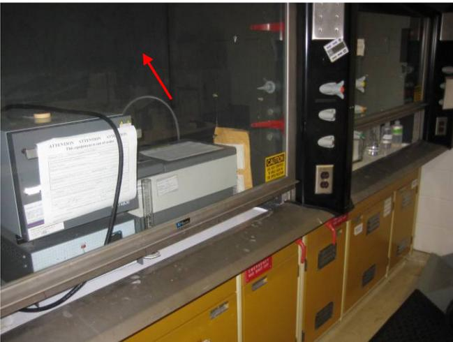
**Photograph 3:** [Room 225] Asbestos-containing Transite cement panels within fume hoods observed to be in good condition.
