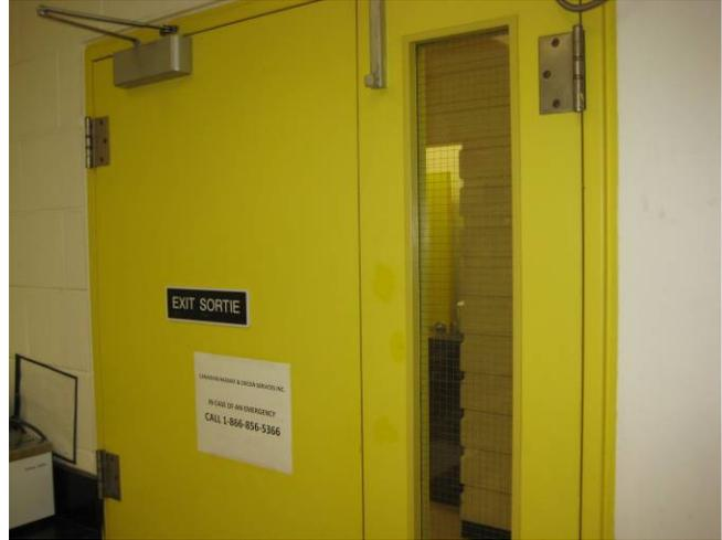
**Photograph 6:** [Room 165] Lead-containing yellow paint application (HC-L3) observed to be in good condition.
