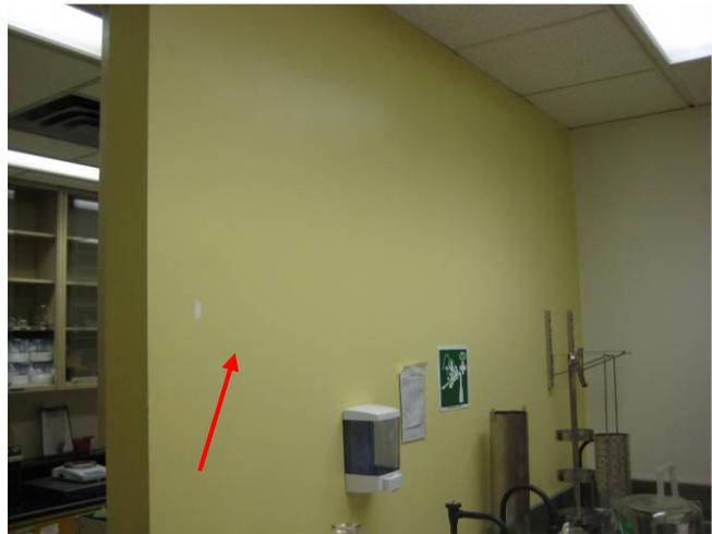
**Photograph 4:** [Room 165] Asbestos-containing drywall joint compound observed to be in good condition.
