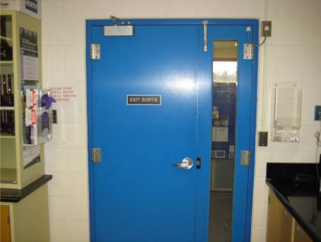
**Photograph 5:** [Room 225] Lead-containing white wall paint application (V-L-06) and blue door frame paint (HC-L1), both observed to be in good condition.
