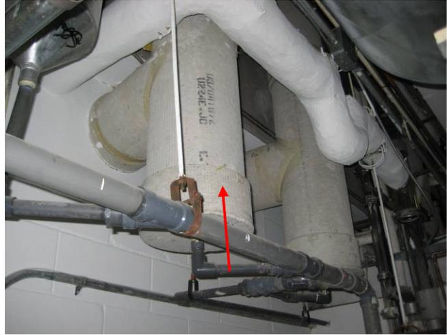
**Photograph 2:** [Service Cores] Asbestos-containing Transite cement piping observed to be in good condition.
