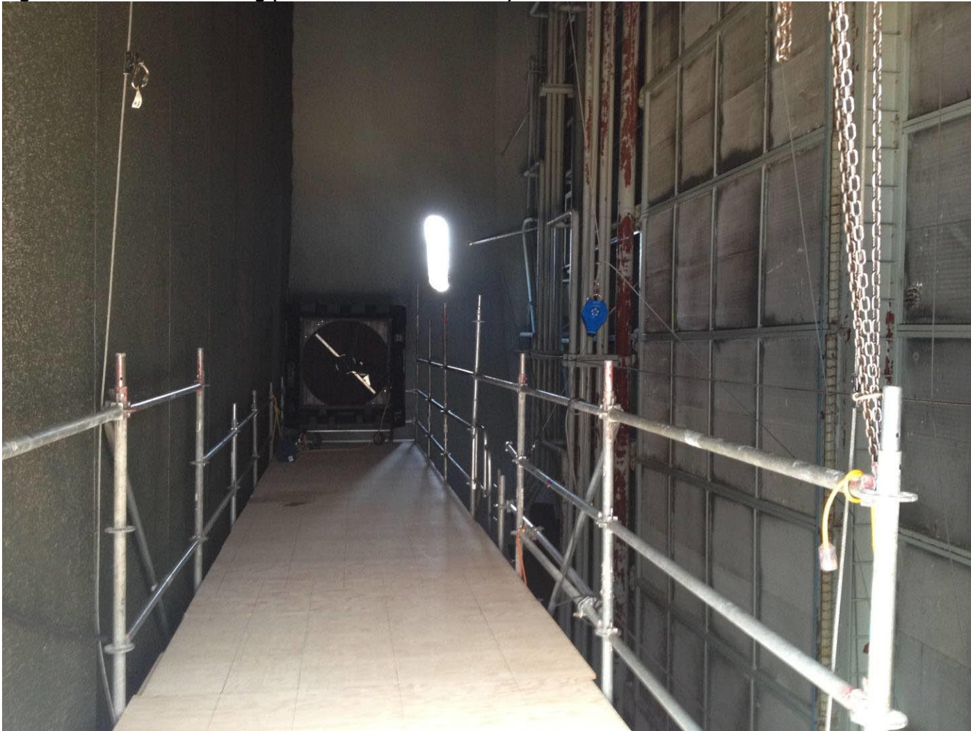
Figure 11: Interior Scaffolding (Mast Climber not Installed)
