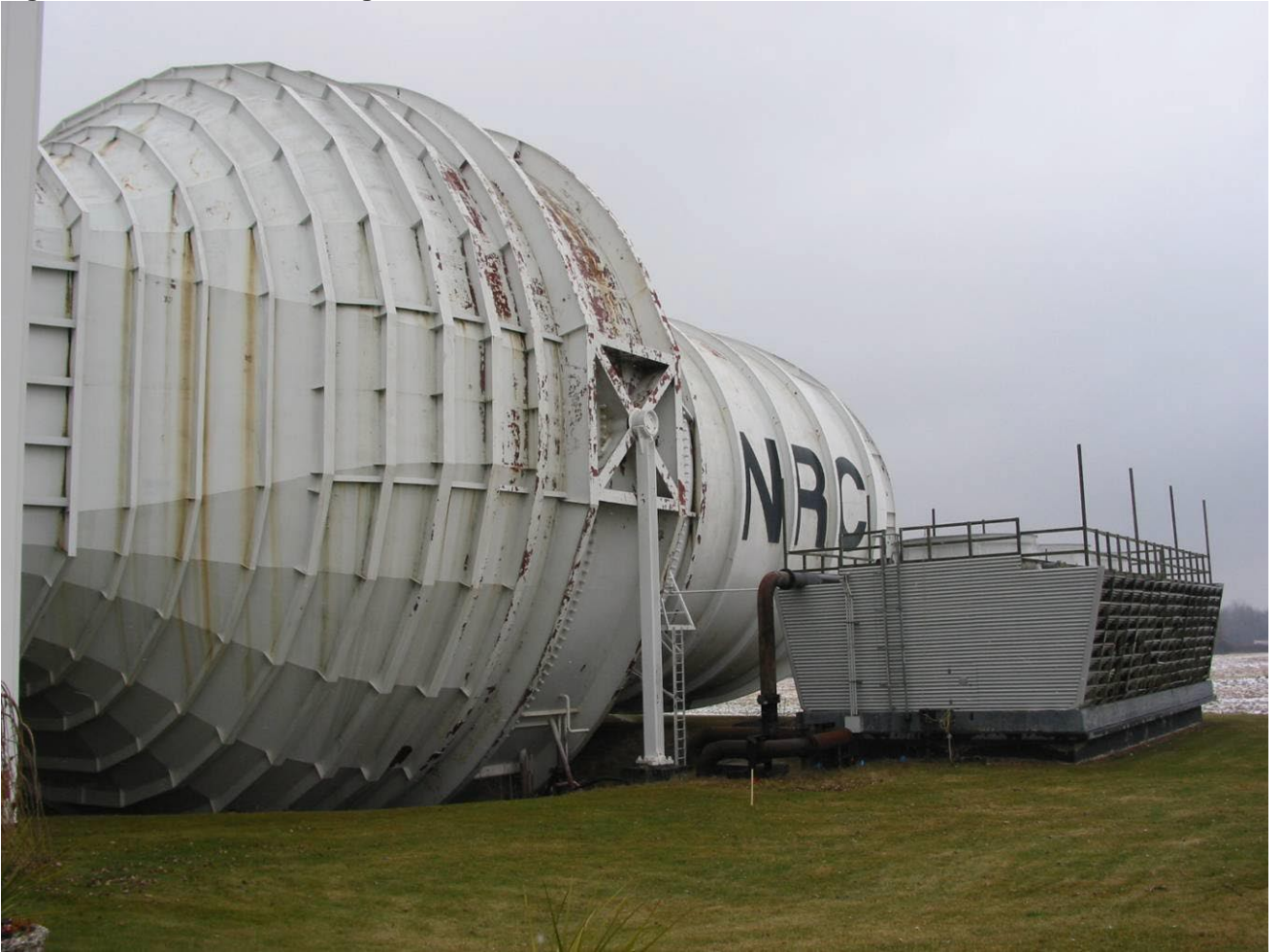
Figure 1: Wind Tunnel Settling Chamber
