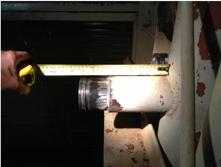
Figure 9: Example of a 3" Grooved Pipe Adapter Ready for Welding to a 3.5" Branch of the 8" Drain Line.
