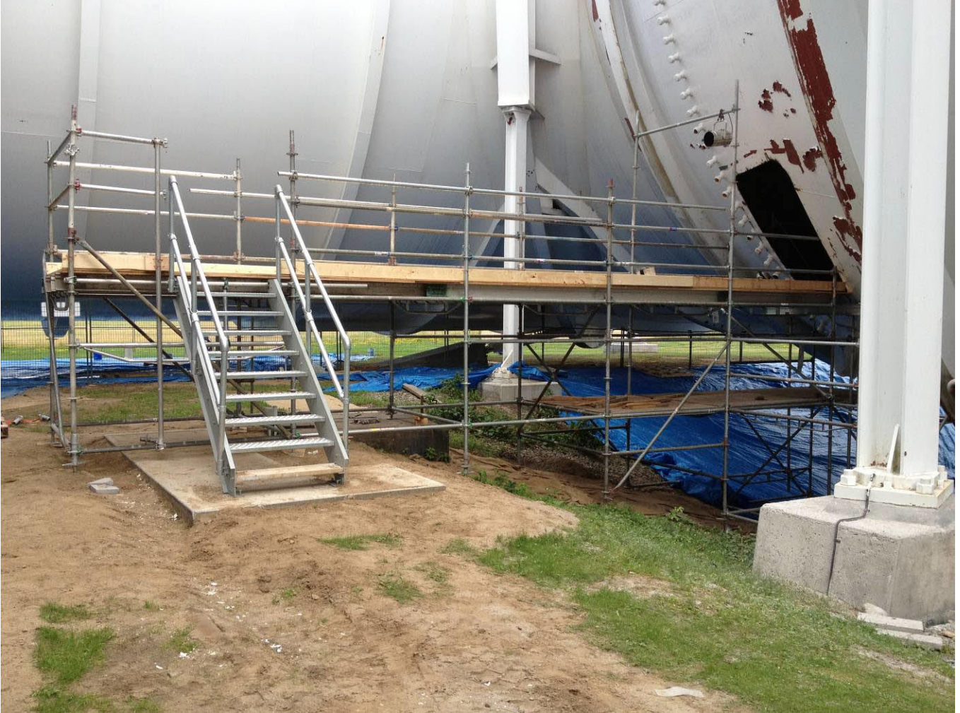
Figure 10: Exterior Scaffolding and Access Hatch
